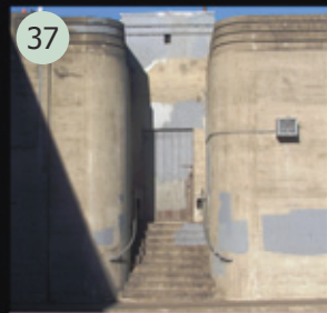
Built: 1935 Style: Streamline Moderne Architect: Unknown
